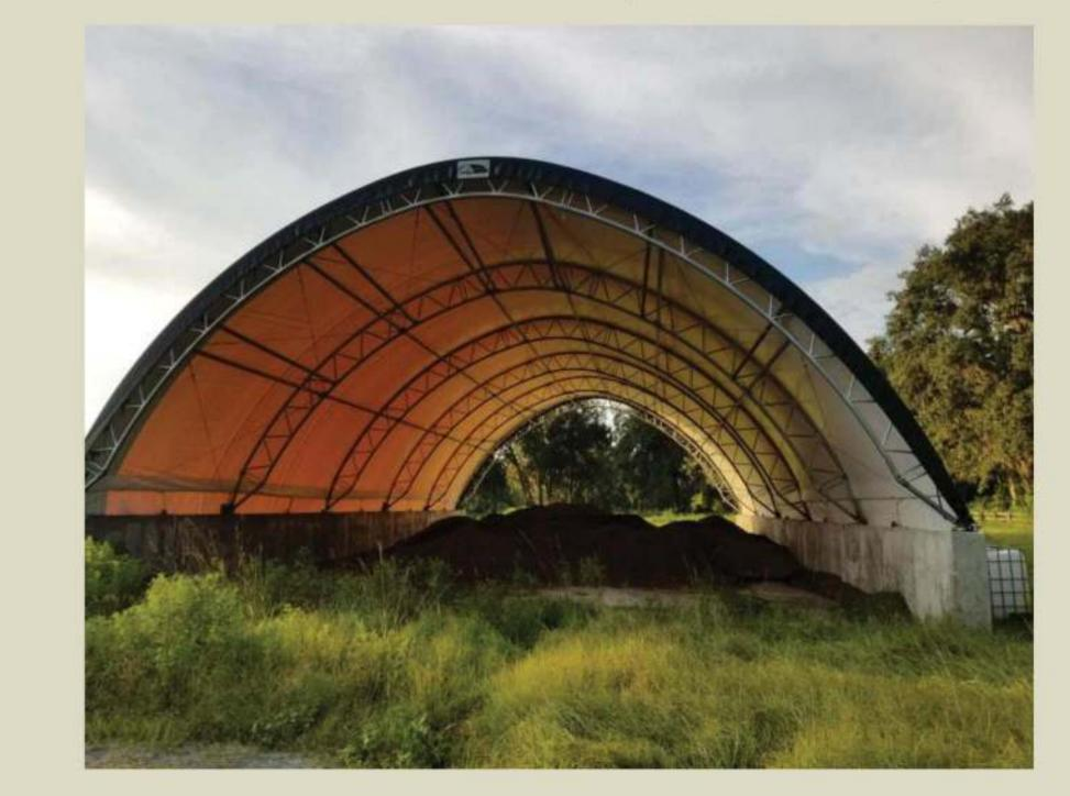
Commercial, prefabricated compost structure that is managed by windrowing manure. A retention pond was dug to the east of the structure to catch any possible runoff.
