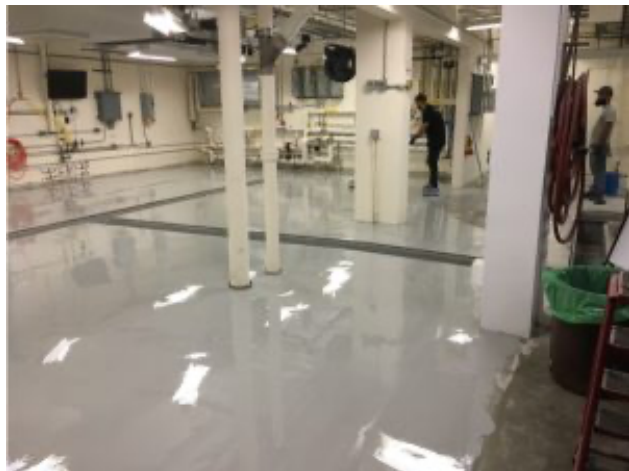
The FSHN Pilot Plant after renovations.
