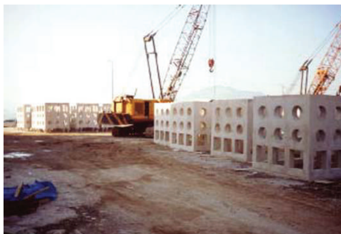
Fig. 10 The box reef design used in Korea resulted from a collaboration of engineers and biologists. Modules have been placed in research plots within Tongyong Marine Reserve for use in experiments with stocking juvenile fishes. Photograph by Kim Chang-gil.
